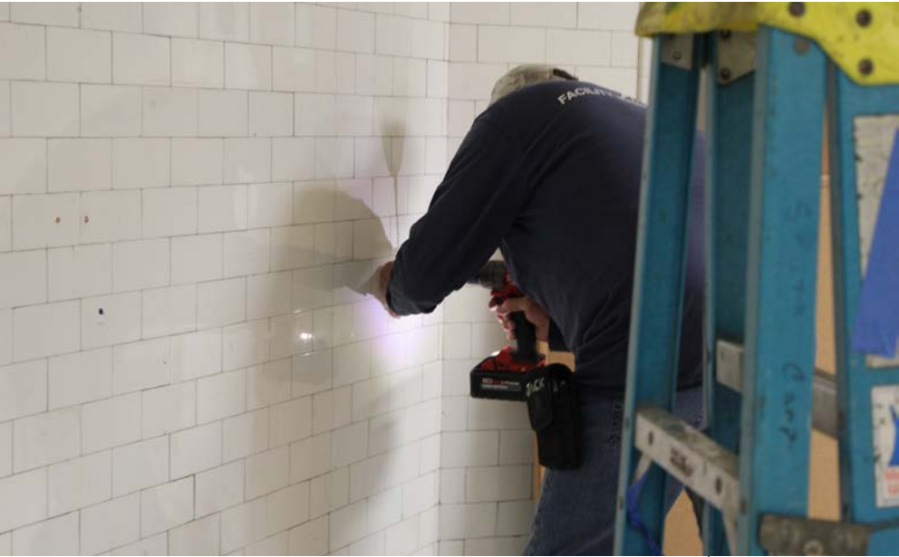
Maintenance drills into basement two side wall. Izabella Kammerer |The Register
